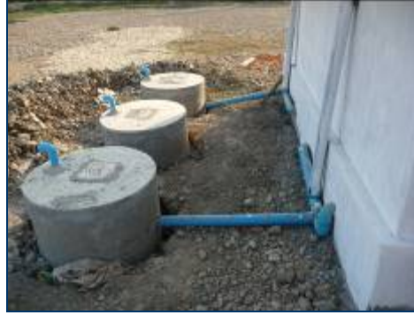
New latrine and septic tanks at Sa U Chaung village in Dedaye Township (Photos from cesvi)
