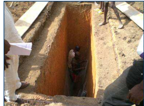
SP, institutional latrine construction (primary school), Lofa County - 2007
