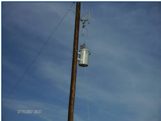
Electrical connection work
