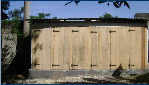
Block of latrines
