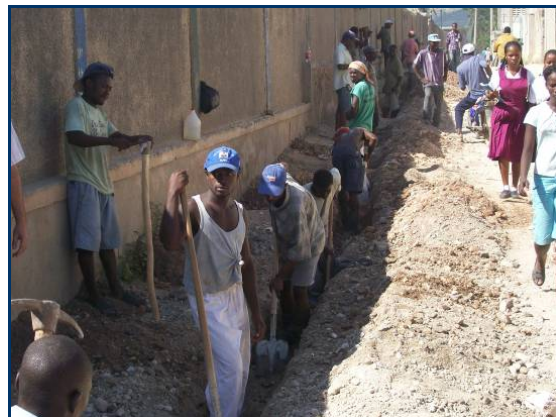
Water connection work
