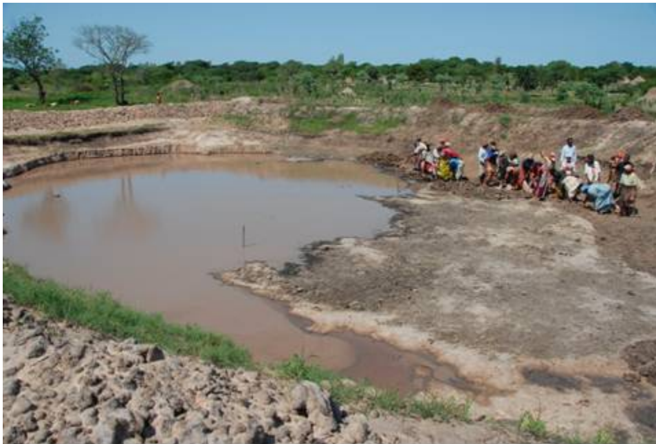
WFP food-for-work project – rain water catchments reservoir – in Moamba District, southern Mozambique. Photo credit: WFP/G. Neuenberg
