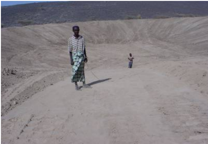
Photo: Construction of a 10,000 m 3 water reserve in Dorra, Djibouti
