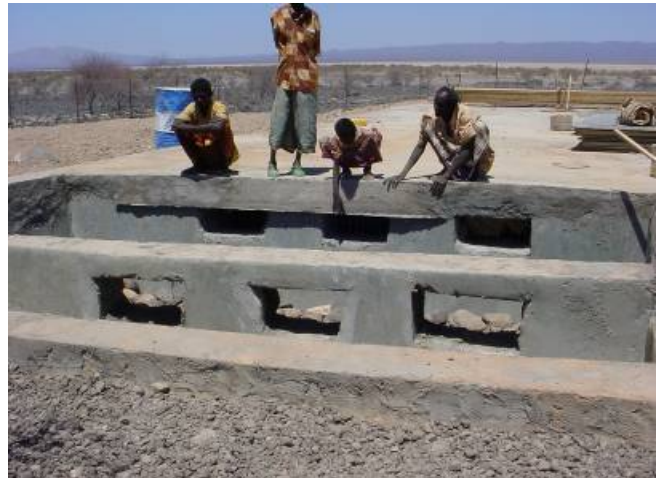
Photo: Construction of a 100 m 3 underground water cistern in Dorra, Djibouti
