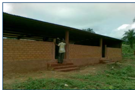
Niplou Town Hall – seen from outside Southern-West (Source : DRC)
