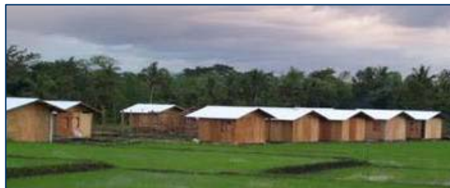
Temporary shelter units in Camarines Sur
