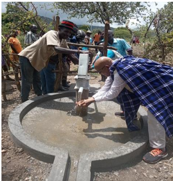
One of the boreholes rehabilitated in Kodonyo village in Kotido district ©UNICEF/2022
