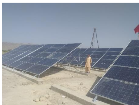
Figure 1: 30KV Solar system installed to pump water from 800 feet deep
